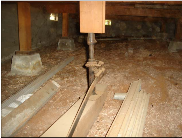
Temporarily supported floor system.
