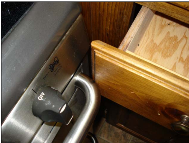
Same problem. New appliances can impede the function of old cabinets.
