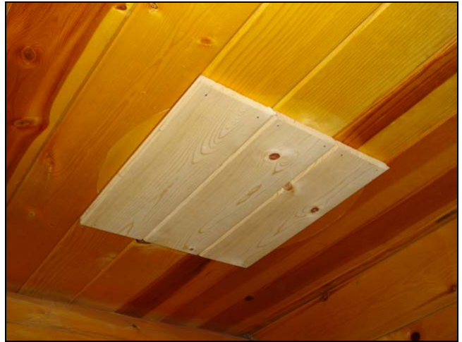
Patching for a former flue pipe.
