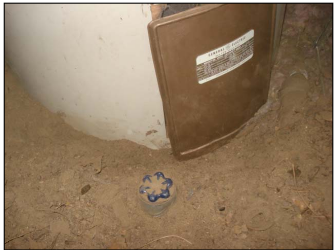
Tank buried in the dirt.
