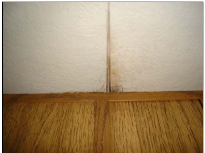
Water intrusion in the acoustical ceiling panels in a manufactured home.
