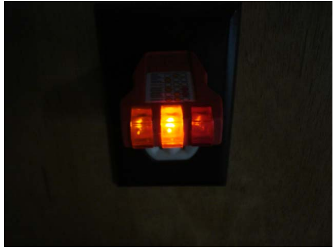
No one ever told me what it means when there appears to be current at all three legs of an outlet, but it can't be good.
