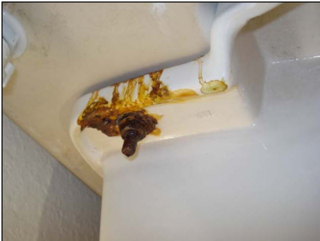
The gasket between the tank and bowl was leaking.
