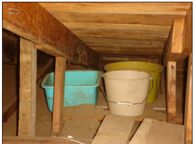
These are custom engineered water collection devices.
