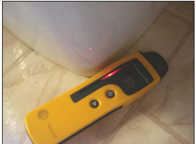
Moisture detector picking up the presence of a water leak from the wax seal. Discoloration was also present. The tool just verifies an active leak.
