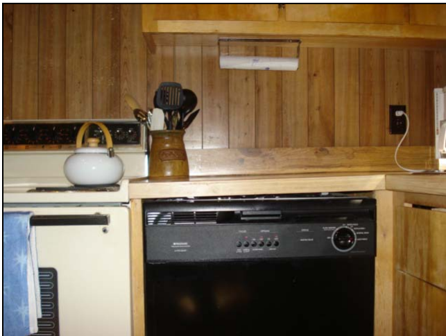
This dishwasher did not fit properly under the cabinet.
