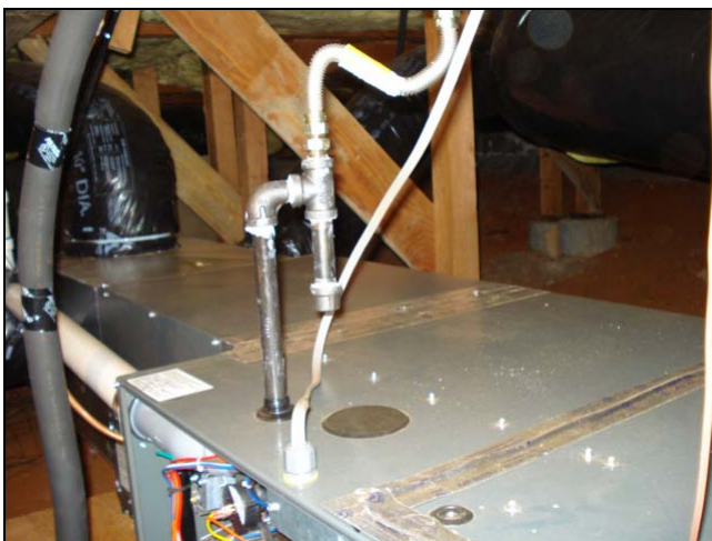
Now that looks good. Kudos to this installer.
