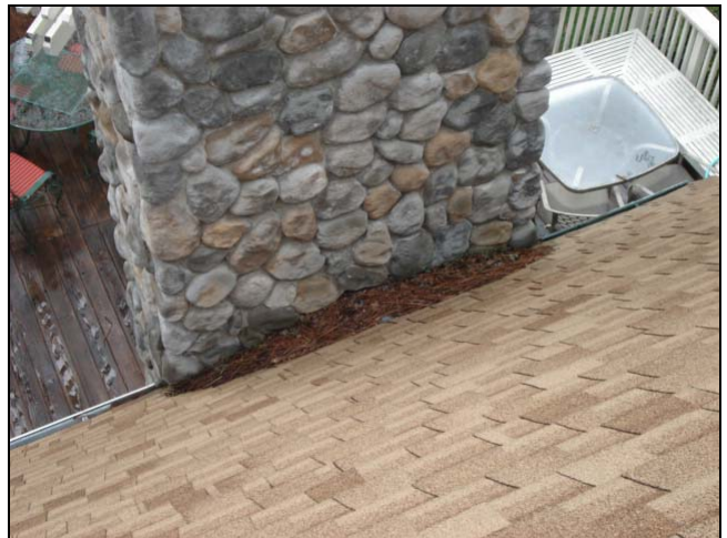
Same chimney, different angle.
