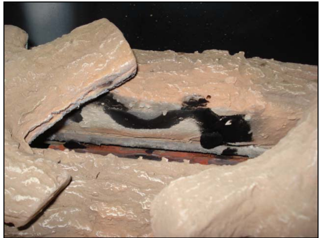
This soot was on a propane gas log and indicates a possible burner or log position needs adjustment.
